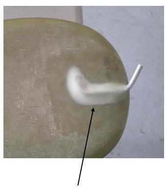
Drilled through existing drain holes into side of tube after tube was mounted and fiberglassed in.
